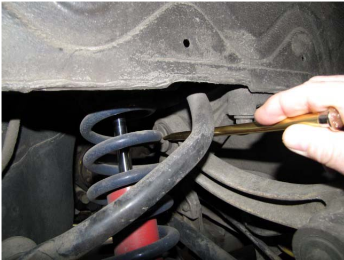
AS VIEWED FROM THE FENDER WELL
